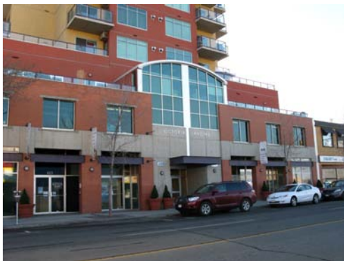
A taller building is more appropriate along a wider, busier street. By stepping back the building at the second or third floor, it retains an appropriate sense of enclosure at street level, while still allowing higher buildings and not overwhelming the street.
