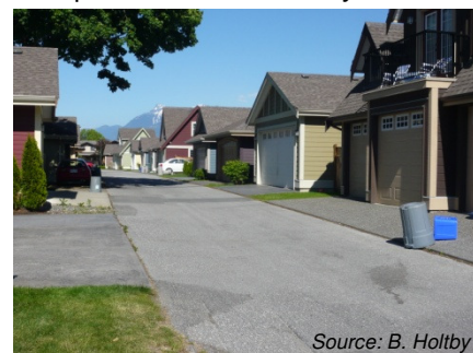
Source: B. Holtby A back alley in a newer development in Chilliwack, BC, featuring shorter driveways and accessory units.
